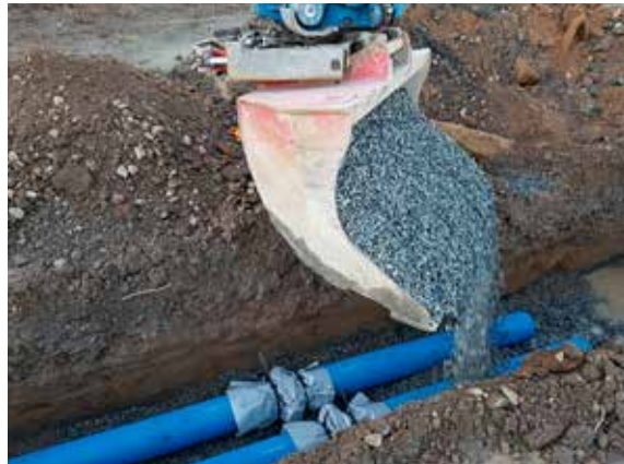
Backfill with 8-16 mm macadam.
